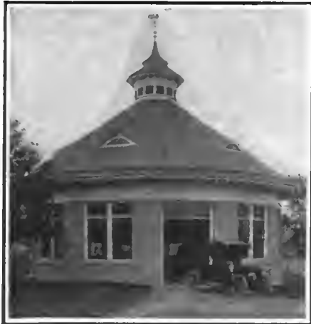
EXTERIOR OF THE CLEMSON GARAGE.
